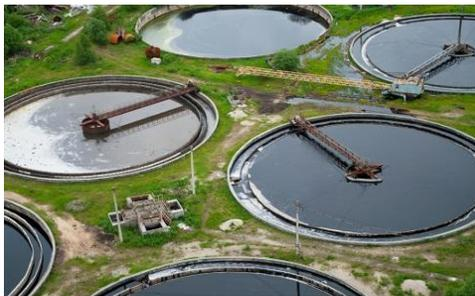
Secondary process consists in a denitrification and nitrification of the water by means of surface mixers and aeration and gravity settling in different tanks by means of pumping.
