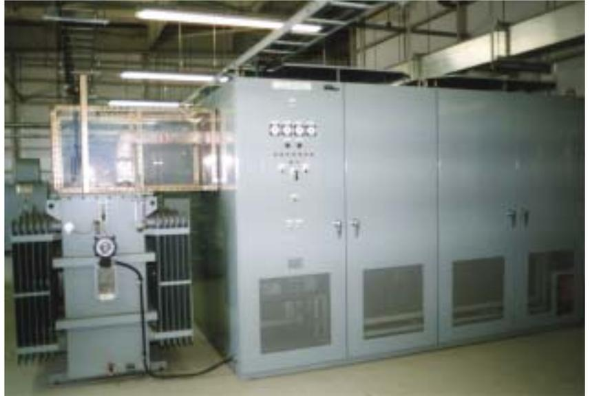
▲ Large-capacity arbitrary-waveform output power supply (FASREC-PW) for aluminum sash coloring
