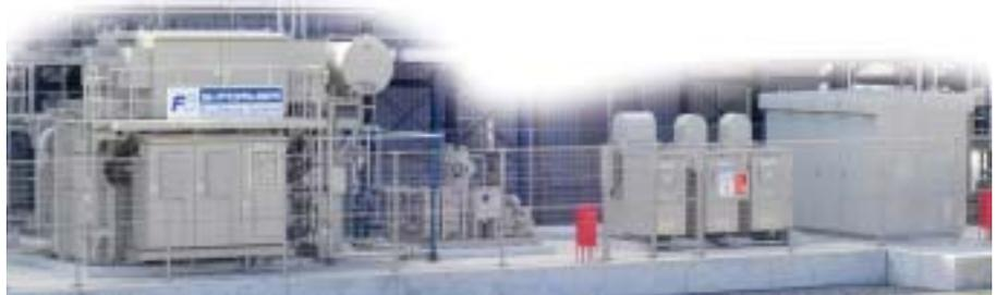
▲ DC power supply for electrolysis (rectifier mounted on top)
