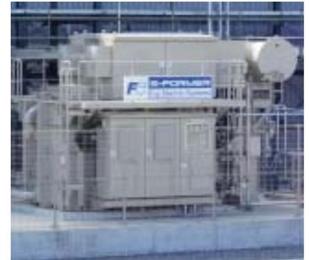
▲DC power supply for electrolysis
